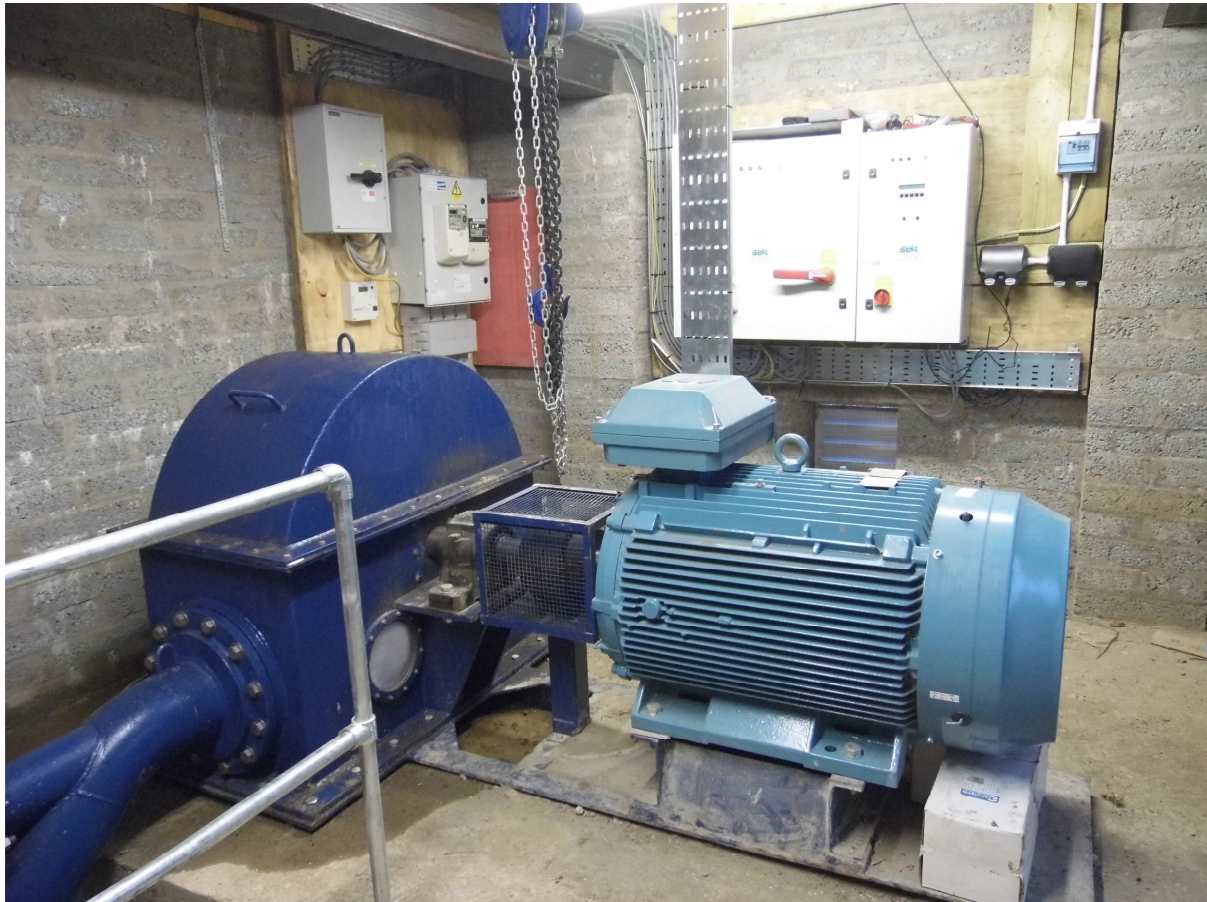
Tepersac Pelton turbine driving 100kW 8 pole generator
